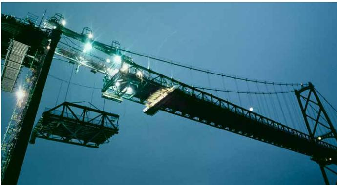
*This photo shows a deck segment being replaced on the Lions Gate Bridge. The same process will be used on the Macdonald Bridge.*
